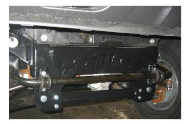
40) Position lower control arms into drop brackets using two  $5/8 \times 5$ " and two  $5/8 \times 6$ " bolts and nuts, DO NOT TIGHTEN at this time.
