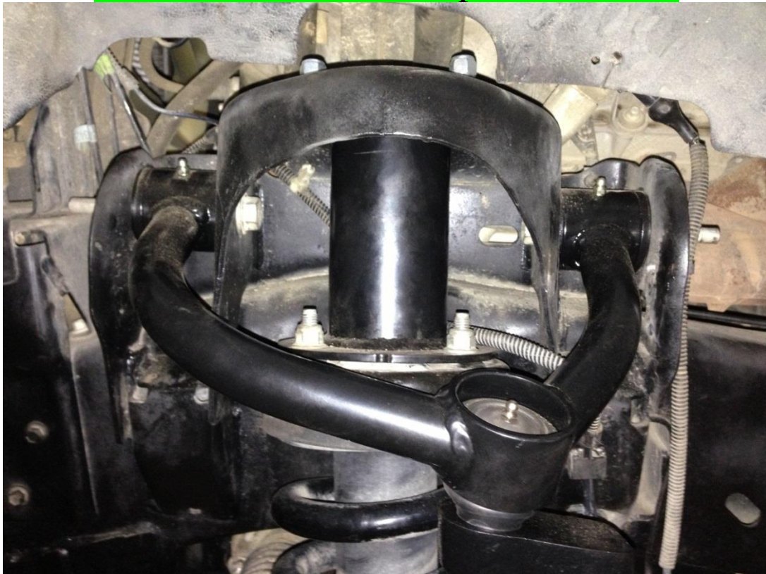
Driver Side Upper Control Arm Installed
